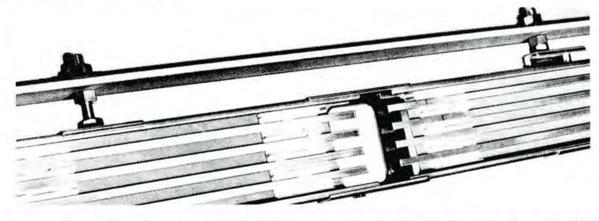
C-shaped trough ends should be joined snugly and wheel bearing surfaces aligned at the joints. Do not displace copper BARS.
